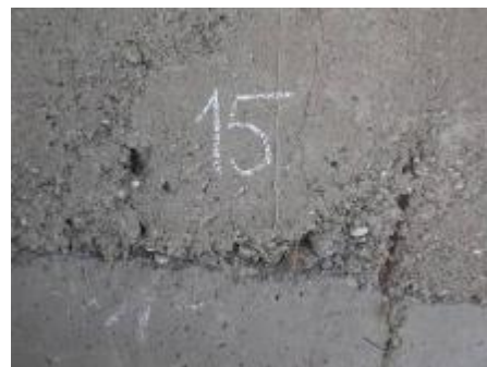
Figure 3. Left: vertical and horizontal crack;; right: concrete segregation zone
