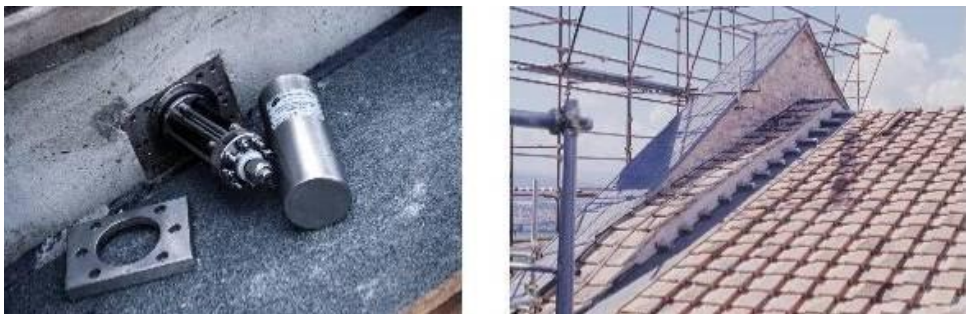
Figure 8. Isolator with SMA seismically favourable connection of the tympanum with the roof of the St. Francesco basilica in Assisi, Italy (2001), [2]
