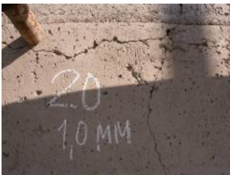
Figure 3. Left: vertical and horizontal crack;; right: concrete segregation zone
