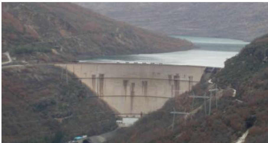
Fig. 19. Grančarevo Arch Dam
