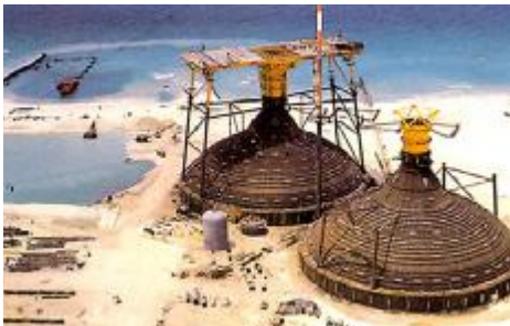
(i) – Construction on shallow dewatered basin on shore
