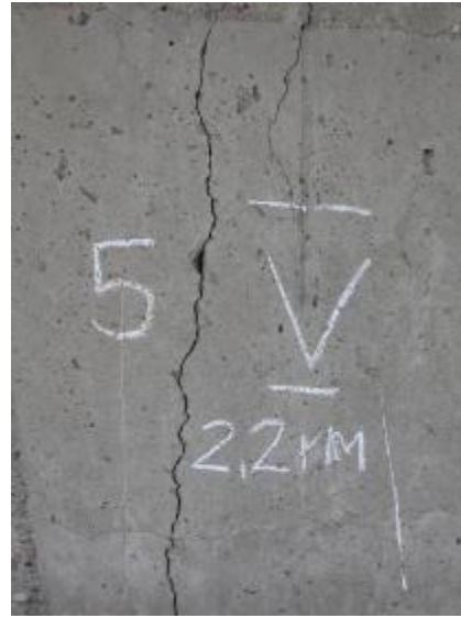
Figure 2. Vertical cracks on the chimney core
