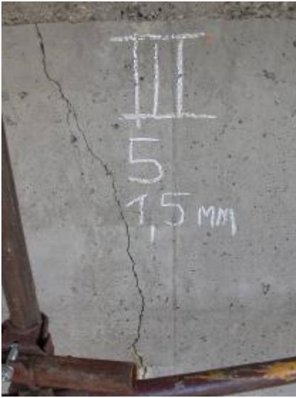
Figure 2. Vertical cracks on the chimney core
