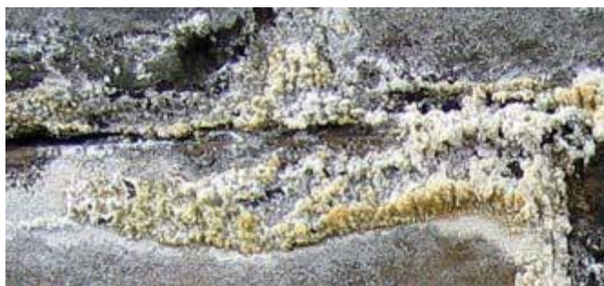
Encrustation – compact, hard, mineral outer layer adhering to the stone. Surface morphology and colour are usually different from those of the stone.
