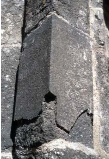
Contour scaling , developing on a magmatic stone element (Kersanton).
