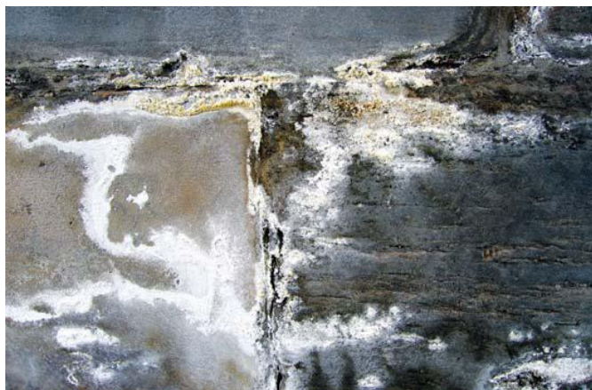
Formation of salts forming efflorescence on the surface of sandstone masonry, focused at joints between masonry blocks.
