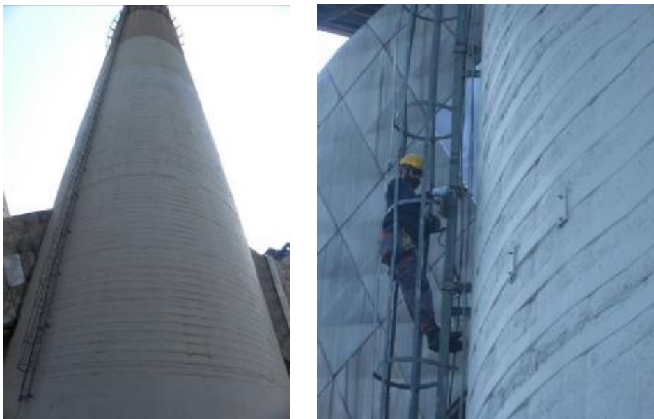
Figure 7. Left: appearance of the part of surface with the glued carbon strips; right: detail of the glued carbon strips, where one of the strip extensions is visible
